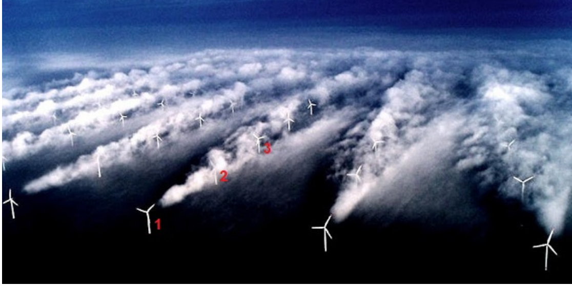
Figure 5: Turbines experiencing multiple wakes. As an example, turbine 3 is experiencing wake effects from both turbine 1 and 2. Image adopted from [4].
